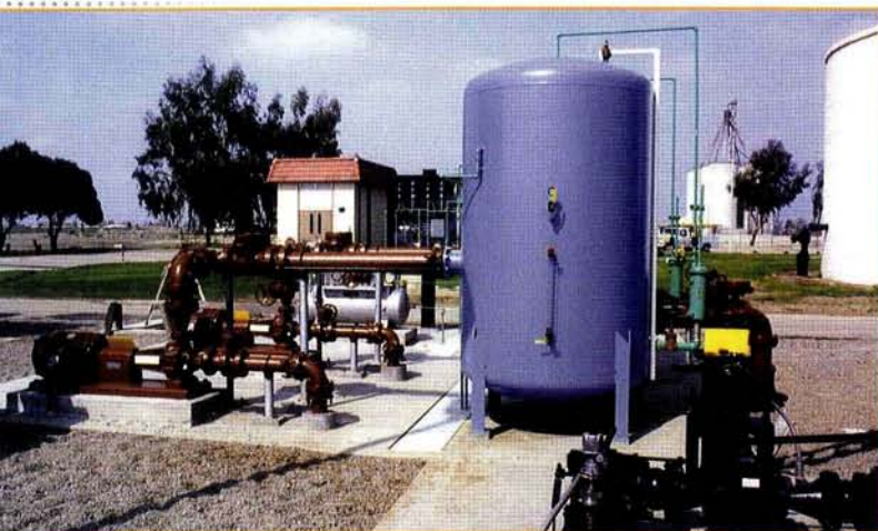
Pressurization system with saturation tank, compressor, air control panel, and pumps
